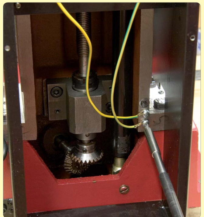
207: Fit earth wires to base of column. Cable tie any loose wires and replace covers
